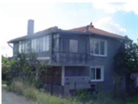
External view of the house
